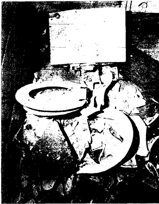
These are some of the sickening sights that confronted Marlyn Koch recently when he checked the buildings at the Wayne County Fairgrounds. The upper photo shows a toilet stool and bowl smashed by a large rock in one of the restrooms, while the bottom picture shows BB holes shot through a windshield of an old car used in parades, which was locked up in a storage building.
